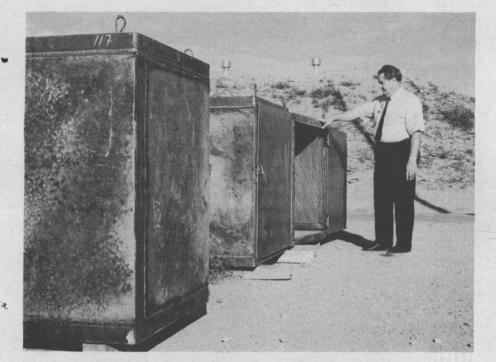
TOUGH CUBES — Lloyd Bonzon (2554) examines explosives storage containers designed for the ECF's on-site storage magazines. Tests have shown that an explosion involving five pounds of explosive material inside one of the cubes will not "sympathetically" detonate explosive materials in a neighboring cube. Each magazine holds up to 24 cubes for a total of 120 pounds of material per magazine. The cubes are made of special fiber-reinforced concrete.
